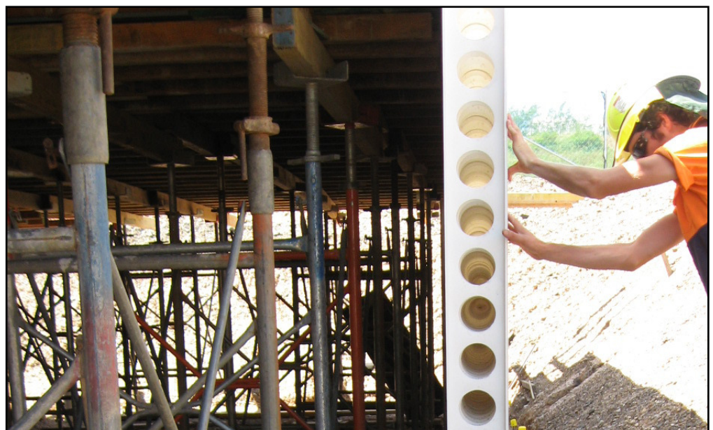
A.W. Edwards uses the Dincel Construction System.
